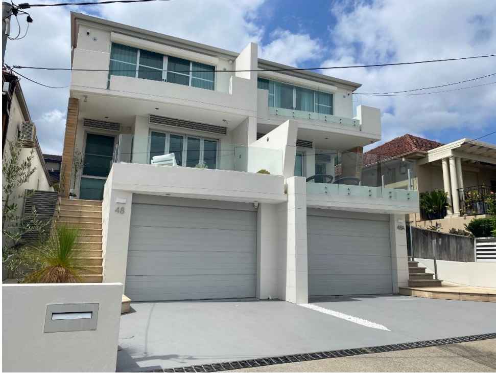
No.48 Woolcott Street, Earlwood
